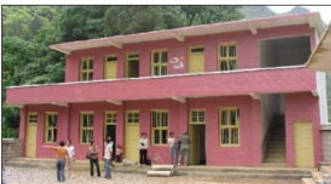
3E's new building for Guxin Primary School
